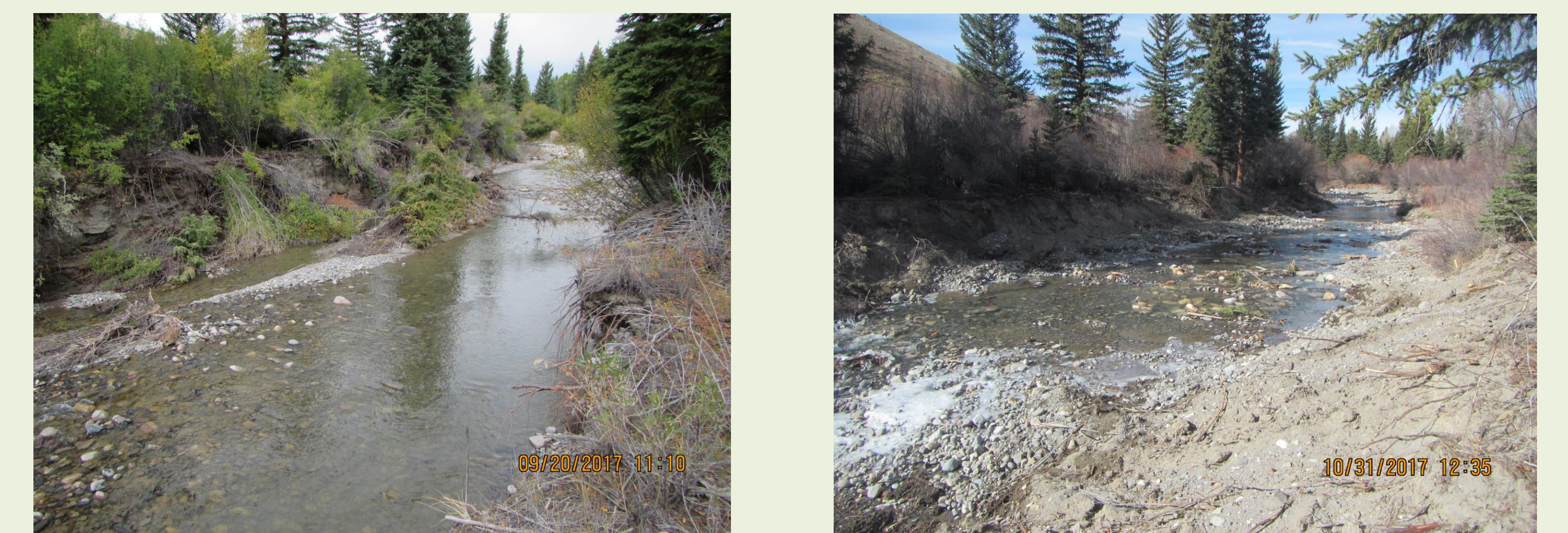
Figure 6. Before (left) and after (right) 2017 constructed riffle installation looking upstream.
