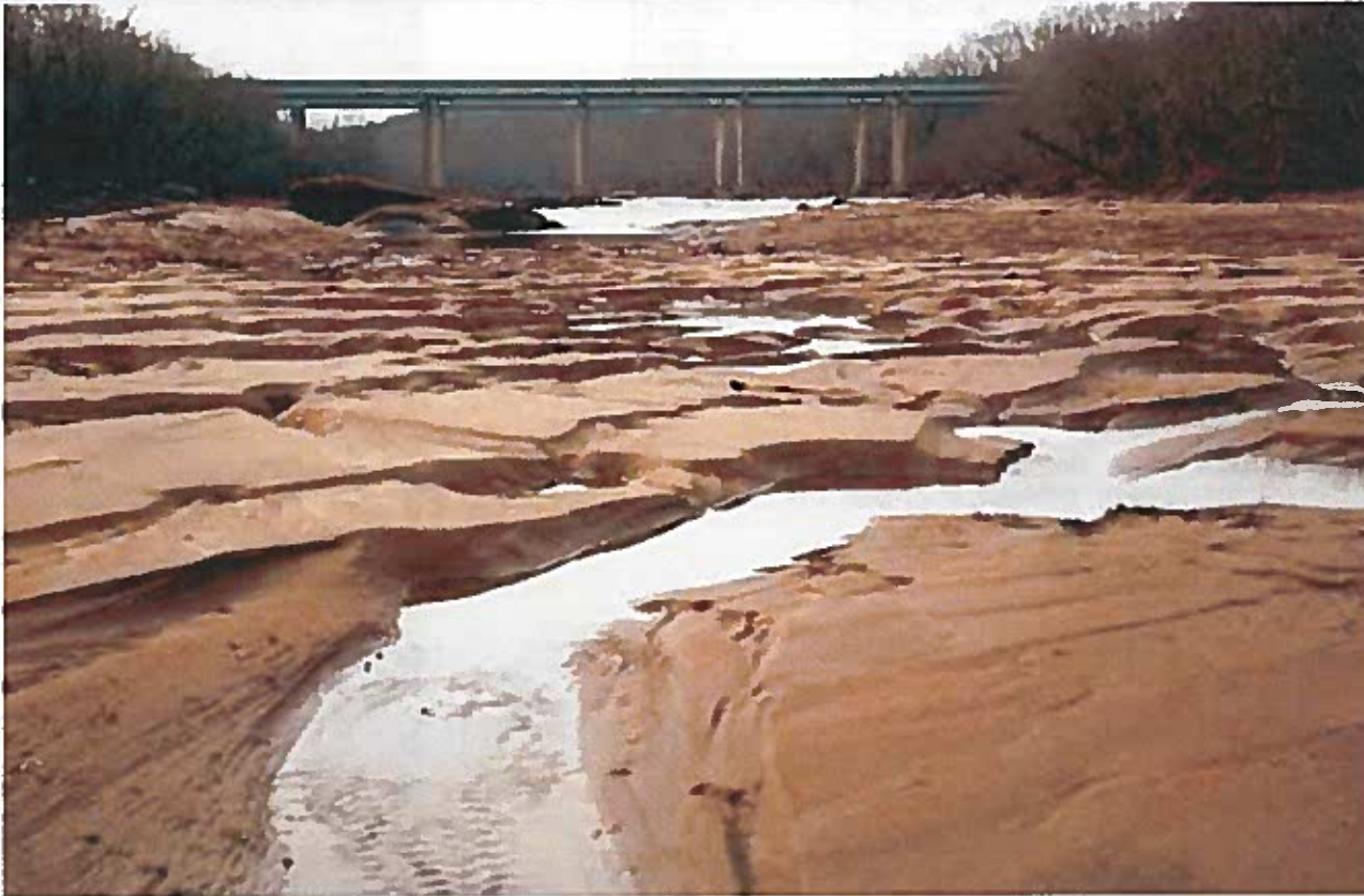
Embrey Dam impoundment following breaching of the dam by the Corps. Dredging was done prior to removal.
