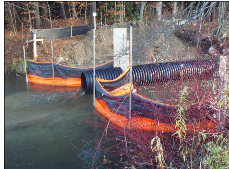
Construction-phase water management
