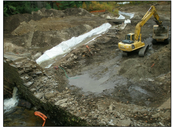
Excavation of impounded sediment
