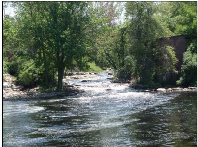
Site of Lower Shannock Dam Removal. Photo by Kristen H. Ferry, IMSG/NOAA Restoration Center.
