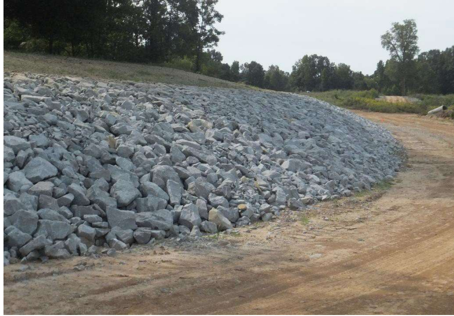
Figure 3 – Shoreline erosion control using rip rap.
