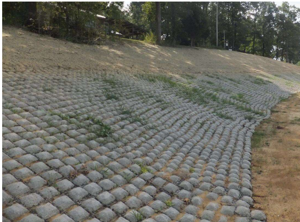
Figure 4 – Shoreline erosion control using Flex-a-mat® fabric.
