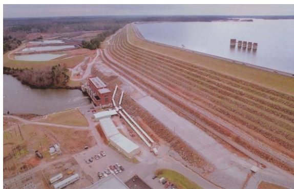
Saluda Dam, impounding the Saluda River in central South Carolina creating Lake Murray, is one of many dams scheduled for relicensing in the next 5 years.
